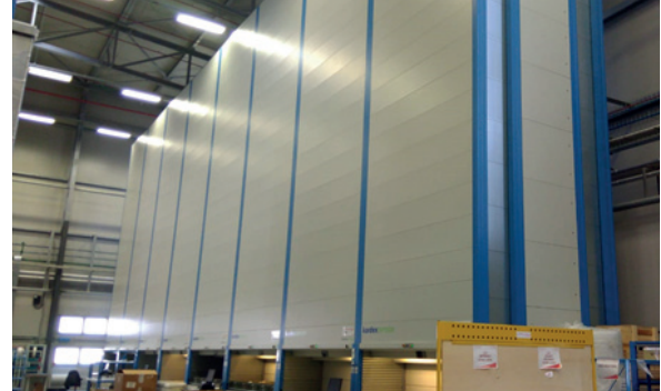
Automated aeronautical parts warehouse
